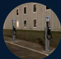
EV Charger Installations on Aecon Properties
