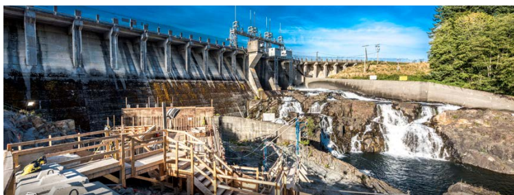
John Hart Generating Station Replacement, BC
